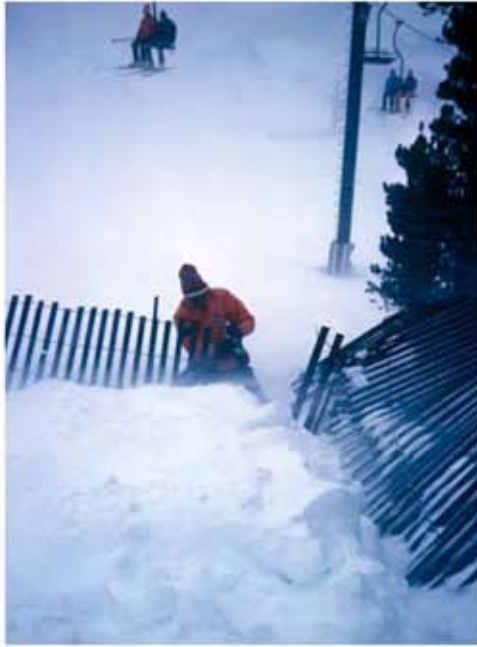
Russ Johnson repairing snowfence, 1976.
