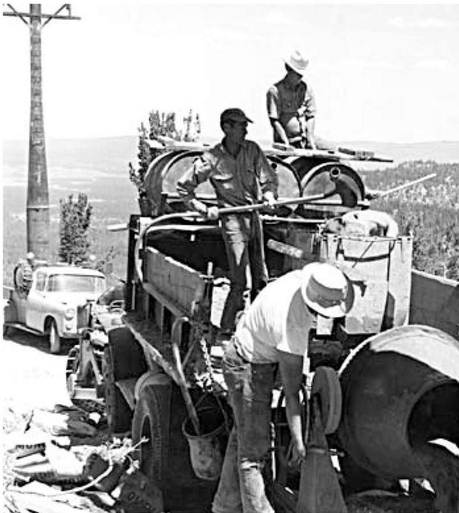
Dave's 4 x 4 GI portable cement-mixer truck that carried sand and gravel in the bed, 150 gallons of water in barrels, and cement bags on top.
