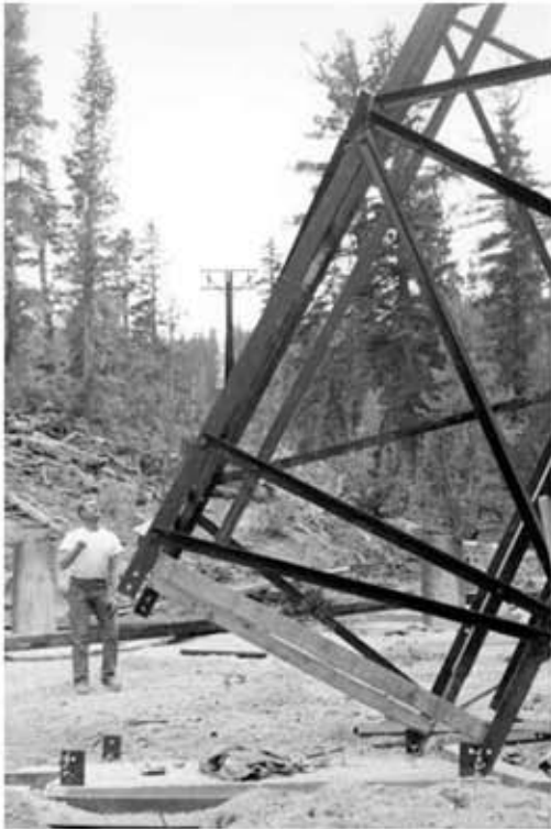
Dave McCoy directing the tower raising for the bottom terminal counterweight.
