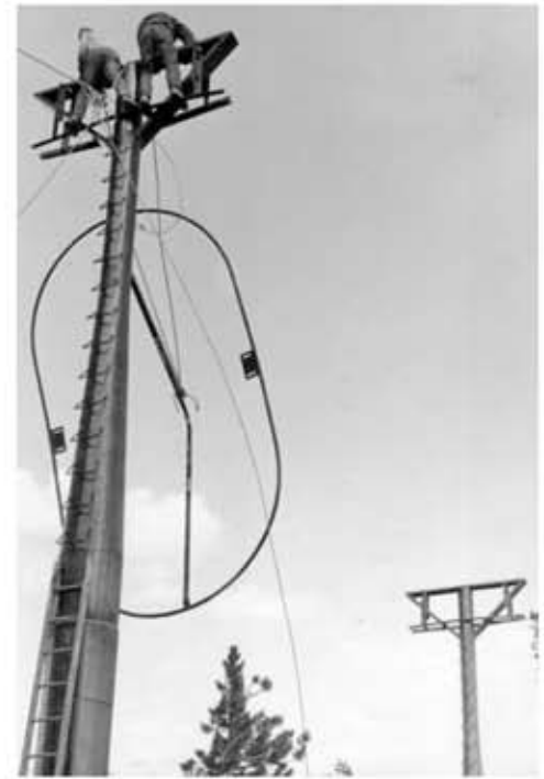
Raising the "halo" guard that kept swinging chairs away from the towers.
