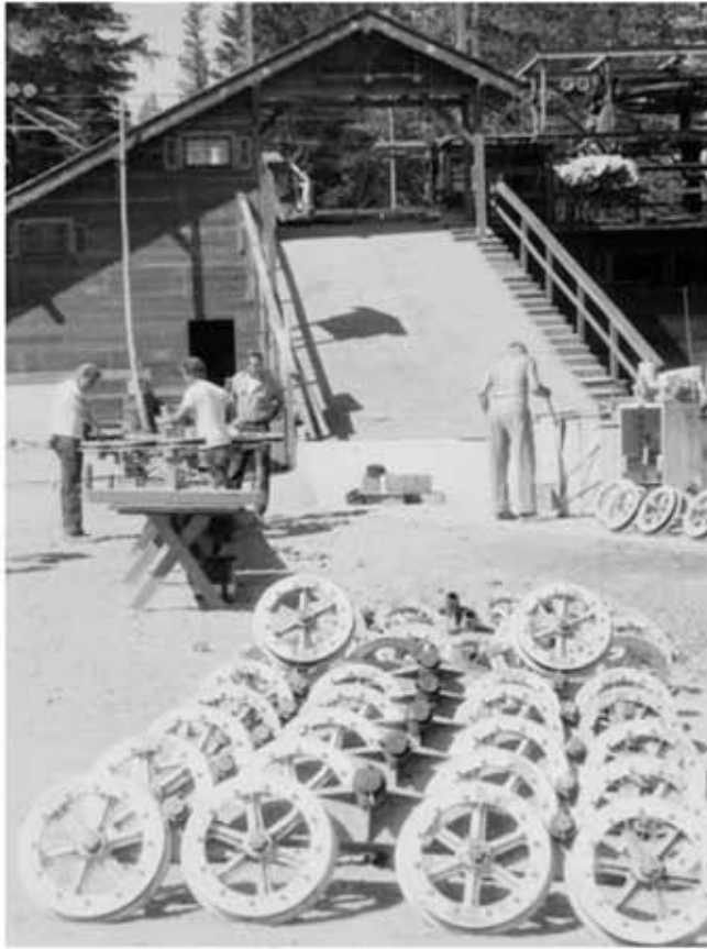
Assembling sheaves at the base of Chair 1 ramp.
