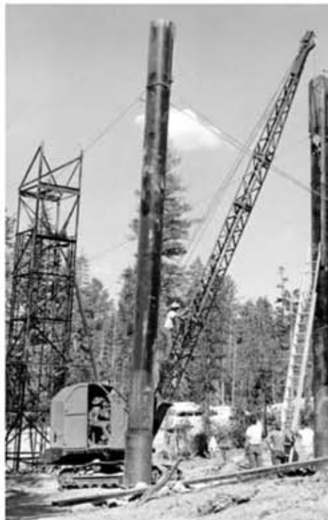
Dave McCoy directing the tower raising for the bottom terminal counterweight.
