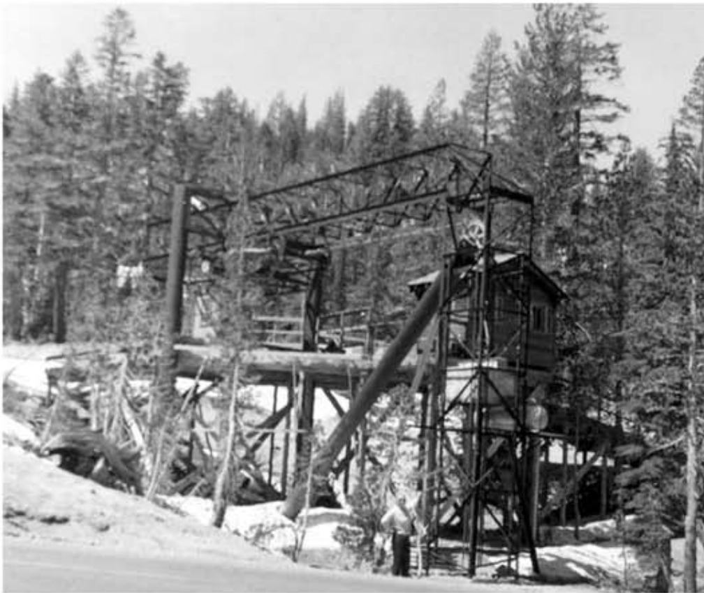
Bottom terminal of Chair 2 with fixed loading zone and a twenty-foot access ramp.
